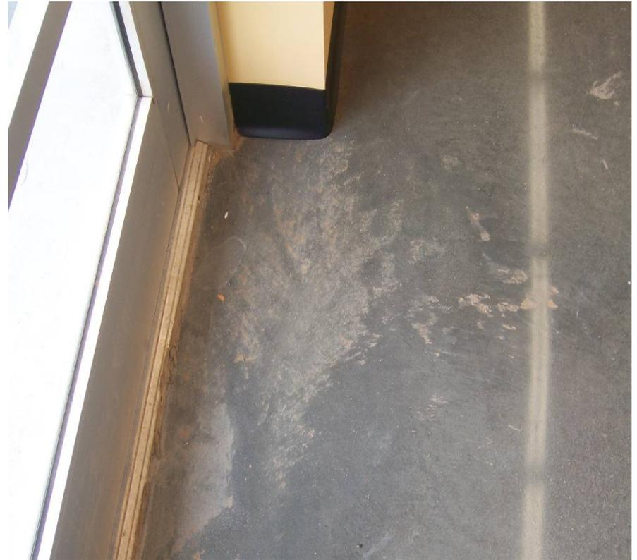
***Poor consolidation cannot be remedied during the grinding / polishing process***
