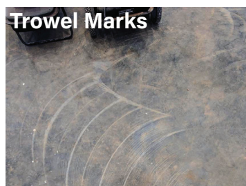
Improper troweling, and using metal blades can burn permanent marks
