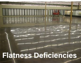
Poor leveling and consolidation results in wavy appearance
