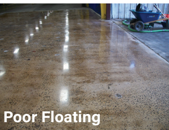
Incorrect placement and floating of aggregate leads to inconsistency
