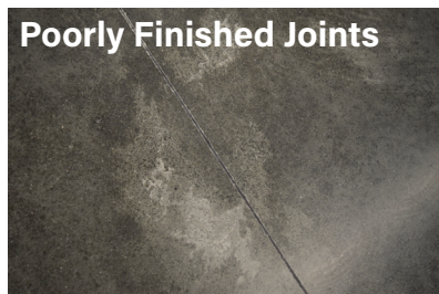
Poorly finished joints resulting in crazing, cracks, and delamination
