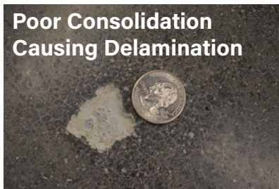
Delamination and voids after grinding due to poor consolidation
