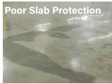
Lack of protection after placement can leave permanent damage
